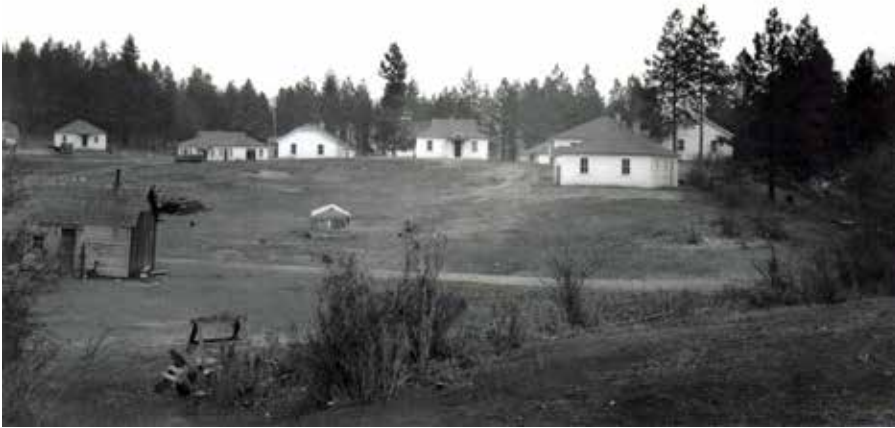
The Kootenai Tribe of Idaho received government housing in 1931 to replace old shacks they were living in. These homes were in horrible condition at the time of the 1974 war. Boundary County Museum Collection
